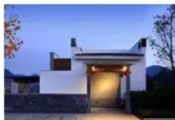
Household Energy Storage
